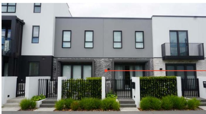
Timber, brick and metal cladding
